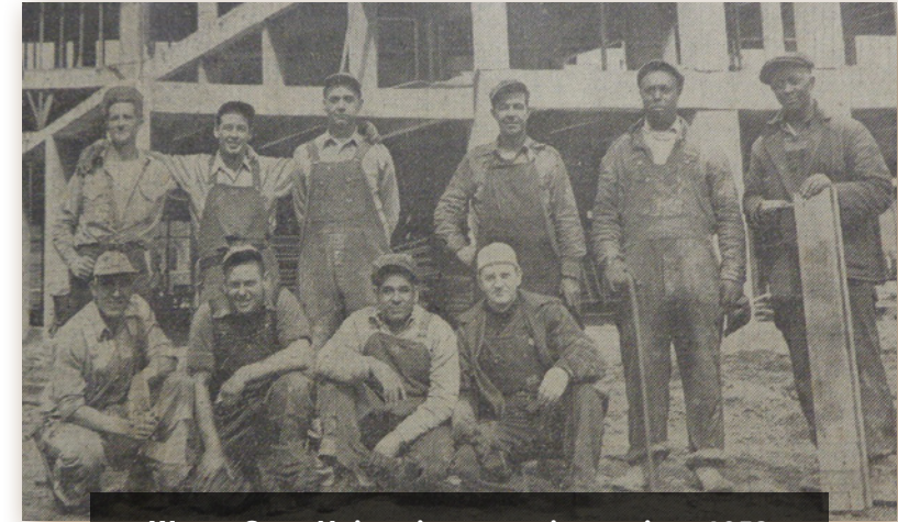
Wayne State University expansion project, 1952
